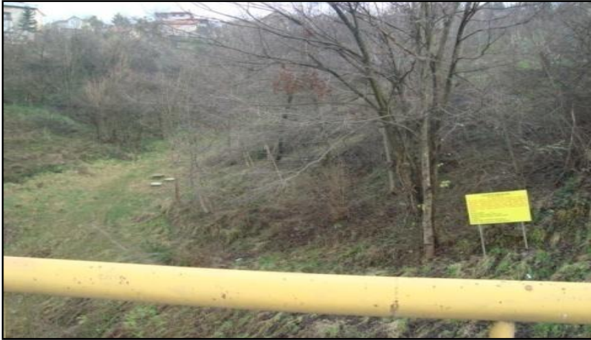
Figure 2: Drainage system and caution board about active landslide in the lower part of Mrakuša locality
