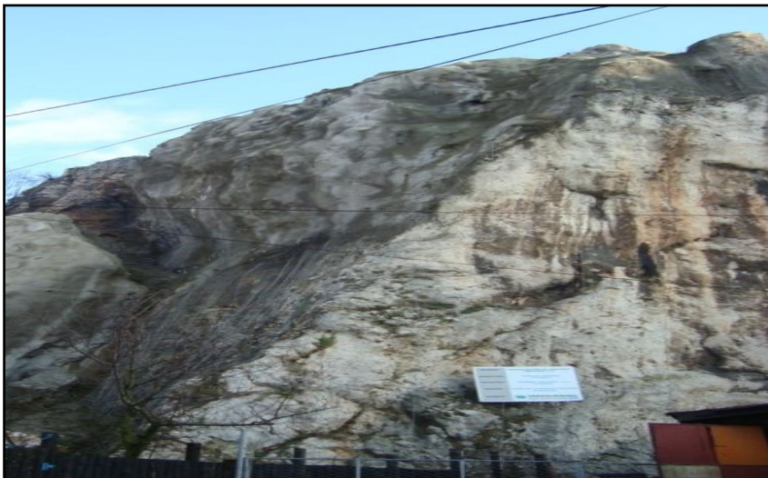
Figure 3: Mitigated escarpment and caution board in the Trebevička Street
